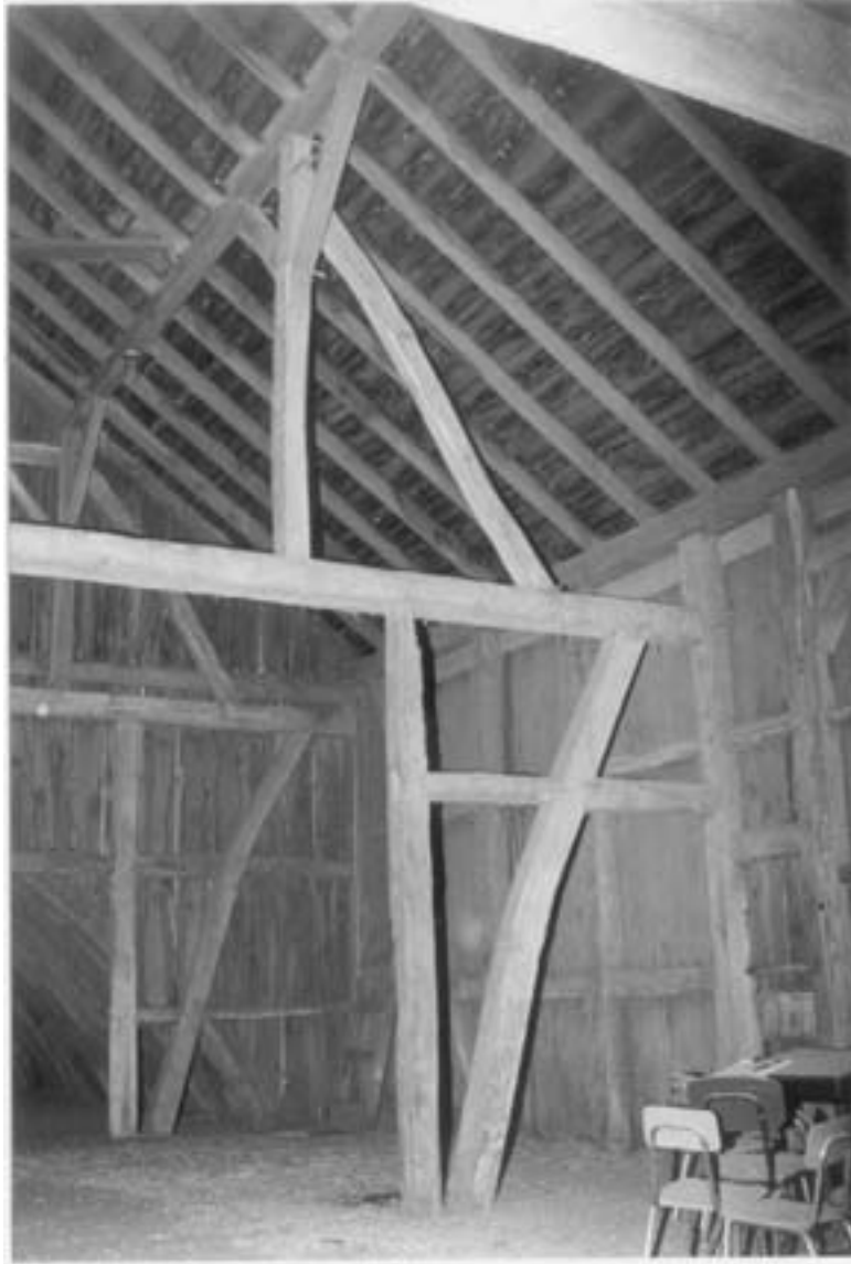
A circa 1880 timber frame barn built on a German immigrant farm in Nicollet County. The barn displays rare Old World construction techniques including plate-to-floor diagonal braces, use of curved timbers, scribed joinery, and fachwerk-style square framing of the exterior walls. Seeman Farm, Courtland Township, Nicollet County, 2005. (Photo by Daniel R. Pratt for Mn/DOT)
