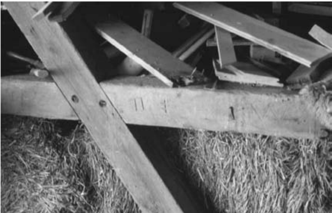
Wooden pegs and carpenter's "marriage marks" in a mortise and tenon timber frame barn built circa 1895 on a German immigrant farm. Dahm Farm, Nicollet Township, Nicollet County, 2006. (Gemini Research photo)
