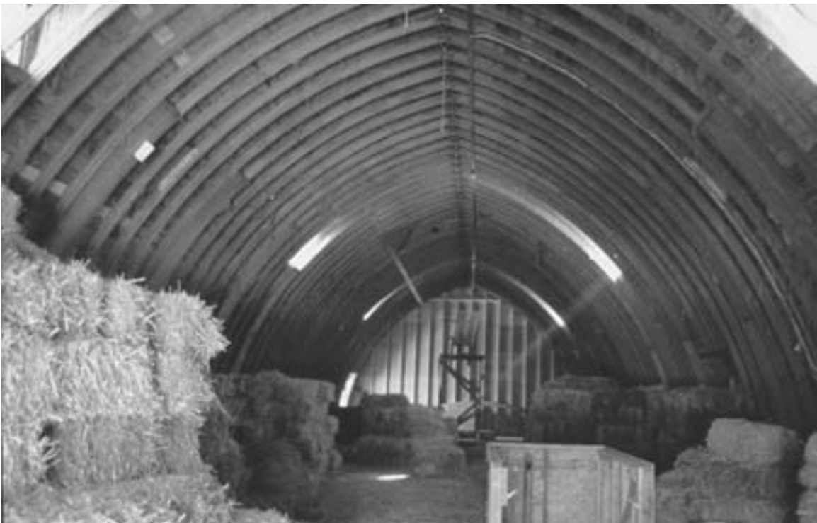
The roof of this gothic arch barn is comprised of a series of glue-laminated rafters made by Rilco in St. Paul. The mow has maximum unobstructed space. West Central School of Agriculture and Experiment Station (now University of Minnesota, Morris), Stevens County, 2004. (Gemini Research photo)
