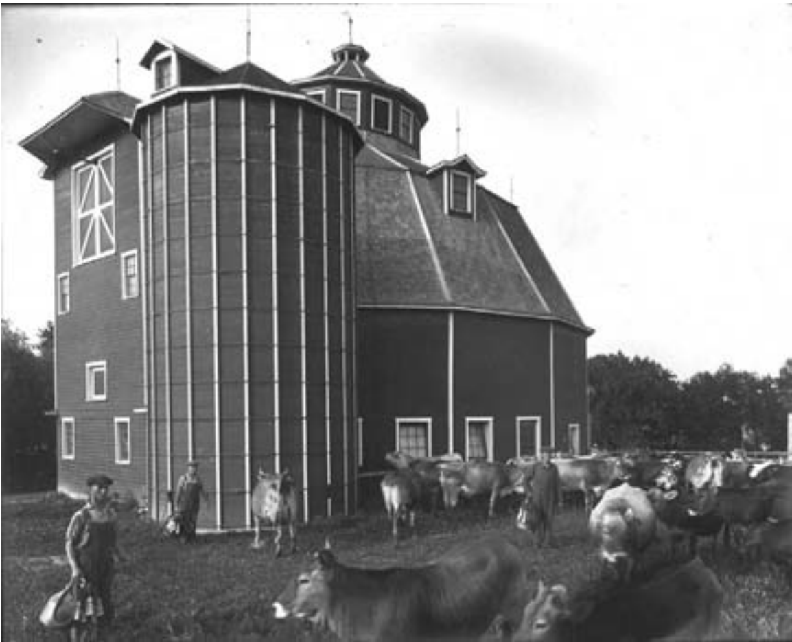
Few farm buildings were designed by professional architects. Instead, beginning in the late 19th century, designs were often influenced by agricultural engineers and other professionals working through colleges, experiment stations, the USDA, the agricultural press, and industry. Location unknown, circa 1910. (MHS photo by Harry Darius Ayer)
