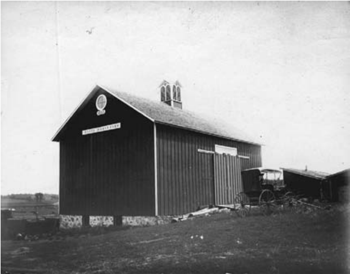
A raised three-bay barn of typical form. It had a gabled roof, central entrance, a long narrow transom window above the door, and few other windows. Placards on the gable end read "1892" and "Hazel Hurst Farm." Location unknown, circa 1900. (MHS photo)
