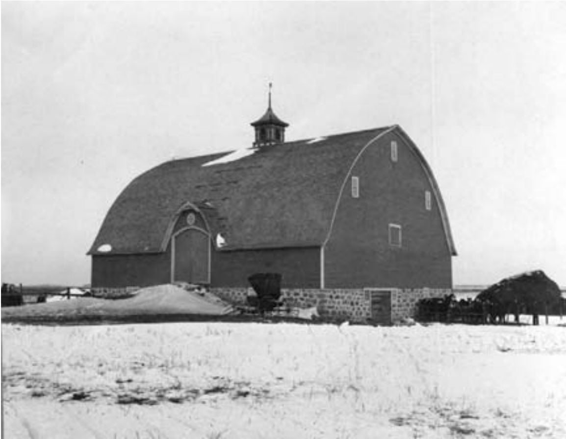
Gothic arches were introduced about 1916. This barn stood in west central Minnesota. Quaal Farm, Lac qui Parle County, circa 1920. (MHS photo by Chalmers and Son)
