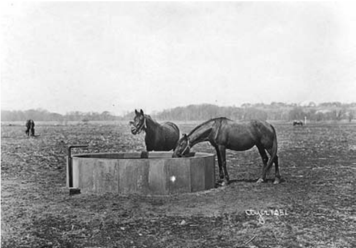
The first cement stave structure in the U.S. was a stock tank built in Michigan in 1905. This photo of a cement stave stock tank was taken circa 1910 on the Savage Farm, presumably in Minnesota (location unknown). (MHS photo by Harry Darius Ayer)
