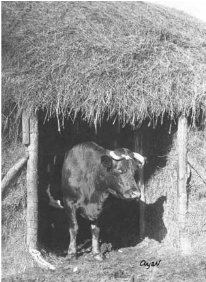
Straw buildings were used in Minnesota for housing all types of livestock and poultry, including shorthorn cattle (shown here). They were built early in the 20th century, during wartime when building materials were scarce, and well into the 1950s. Photo location unknown, circa 1910. (MHS photo by Harry Darius Ayer)
