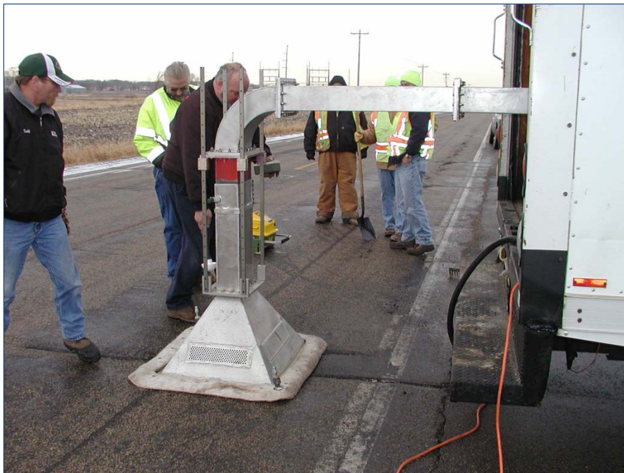
Figure 8. Microwave Pothole Patch Repair
