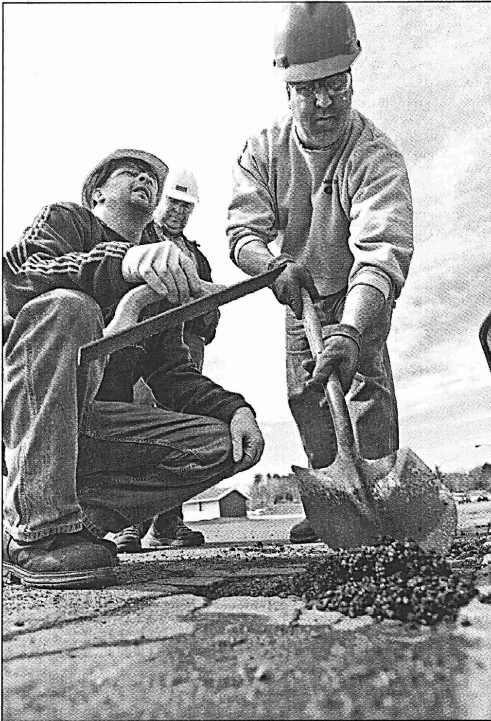
NRRI Coleraine Minerals Research Laboratory technicians Tim Kemp (left) and Greg Gargano, both of Hibbing, fill a pothole in Coleraine with a mixture containing tailings from the taconite mining industry. The pothole mixture is much more dense and durable than conventional asphalt products.
