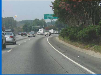
The exit diverge point is hidden by the horizontal curvature and roadside vegetation.
