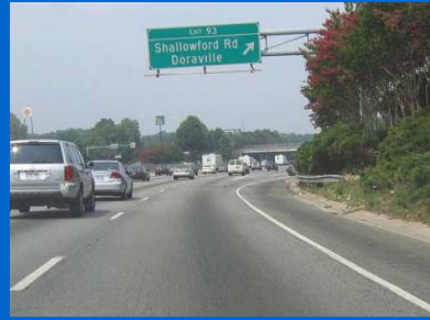
When the diverge point becomes visible, there is little time to adjust for speed and path change (further complicated by a taper style exit on horizontal curve).
